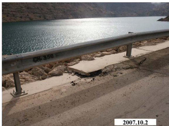
Figure 13. Cracks in the dam crest of Masjed-Soleyman dam
