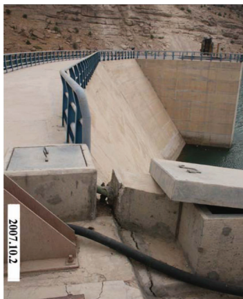
Figure 13. Cracks in the dam crest of Masjed-Soleyman dam
