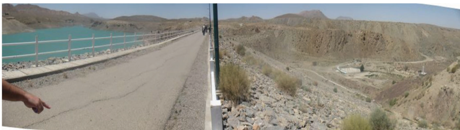
Figure 14. Bumpy crest of Masjed-Soleyman Dam due to non-homogeneous vertical deformations
