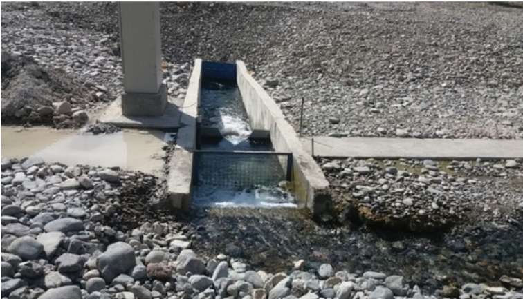
Figure 3. A view of the V-notch seepage control in Silveh dam
