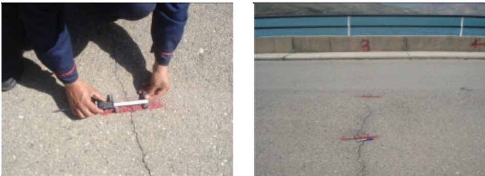
Figure 5. Numbering and monitoring of cracks in the crest of Mahabad dam
