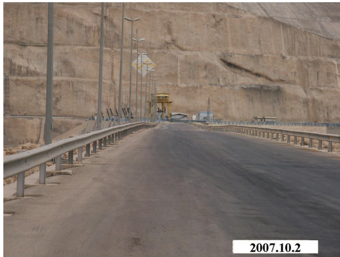
Figure 14. Bumpy crest of Masjed-Soleyman Dam due to non-homogeneous vertical deformations
