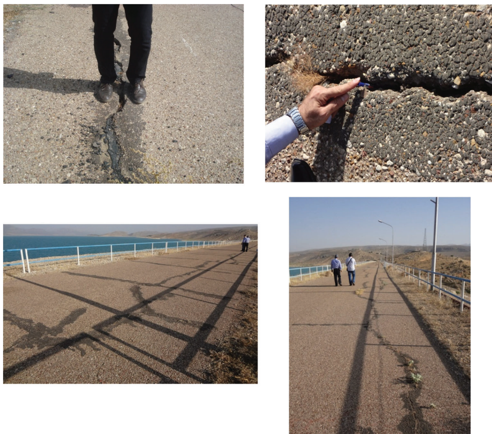
Figure 9. Cracks in crest of Doroodzan dam
