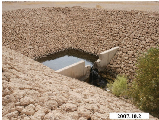
Figure 12. Measuring weir of Masjed-Soleyman dam
